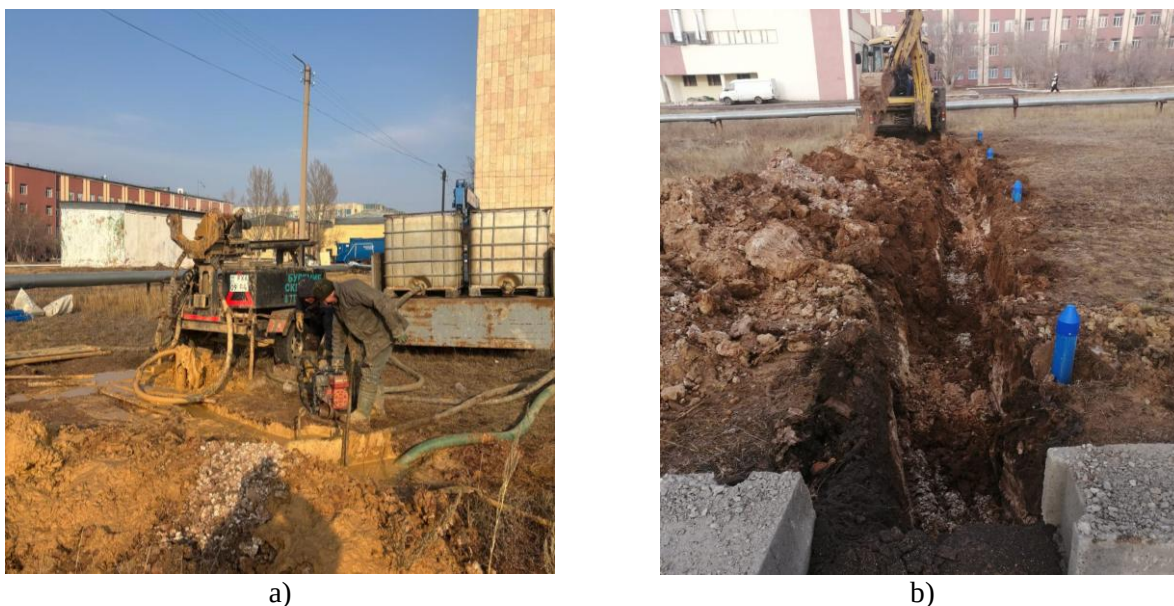
Fig.1. Ground-source heat pump experimental site: a) general view of borehole drilling; b) blue markers indicate boreholes along the trench.
