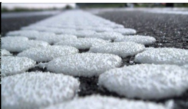
Fig. 6. Glass bead coating.
