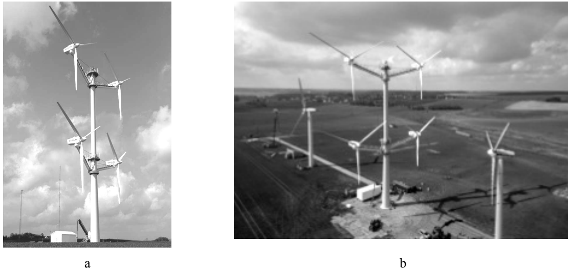
Fig.3. «Vestas» multi-rotor wind farm: a) main view of a 4-rotor wind turbine; b) experimental wind turbine test farm [9].
